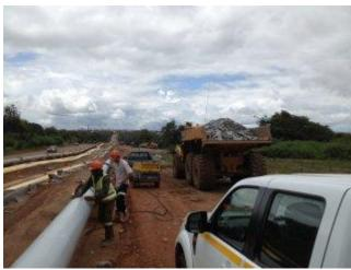
South Africa-based pipeline solutions provider Rare is working on a R6.3-million infrastructure contract for steel piping, which conveys abrasive and corrosive mining slurry from the plant to the tailings dam, for Zambian copper mine Kansanshi.
