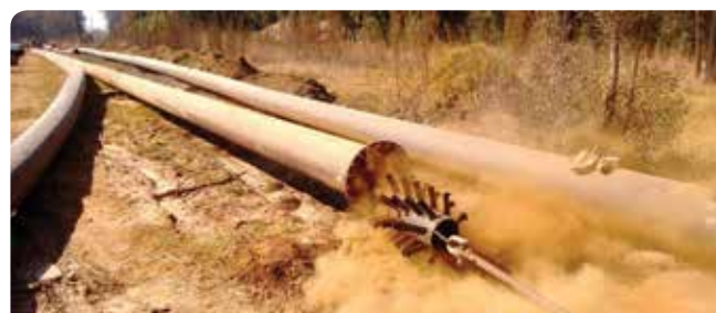
BELOW This existing pipeline is being prepared to be lined in situ with HDPE liners, offering a significant cost advantage
