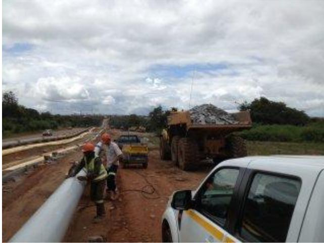
South Africa-based pipeline solutions provider Rare is working on a R6.3-million infrastructure contract for steel piping, which conveys abrasive and corrosive mining slurry from the plant to the tailings dam, for Zambian copper mine Kansanshi.
